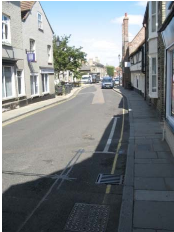
Parking removed from Kneesworth Street approach to The Cross, to allow buses room to pass through
